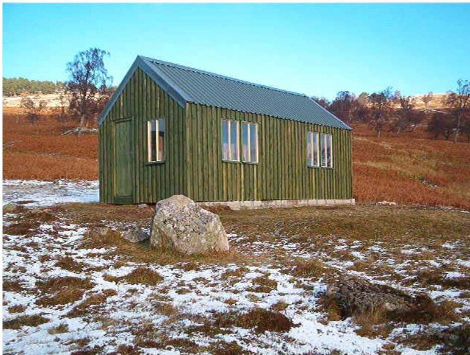
Fig 2 Shelter for retention
